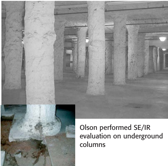
Performing SE/IR evaluation on concrete foundation walls
