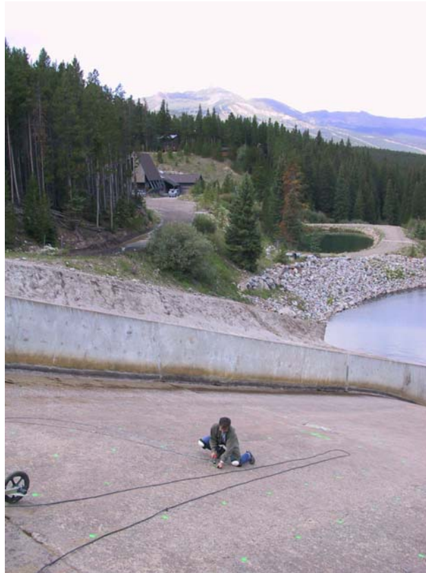
Figure 1.: Overview of the alpine dam spillway
